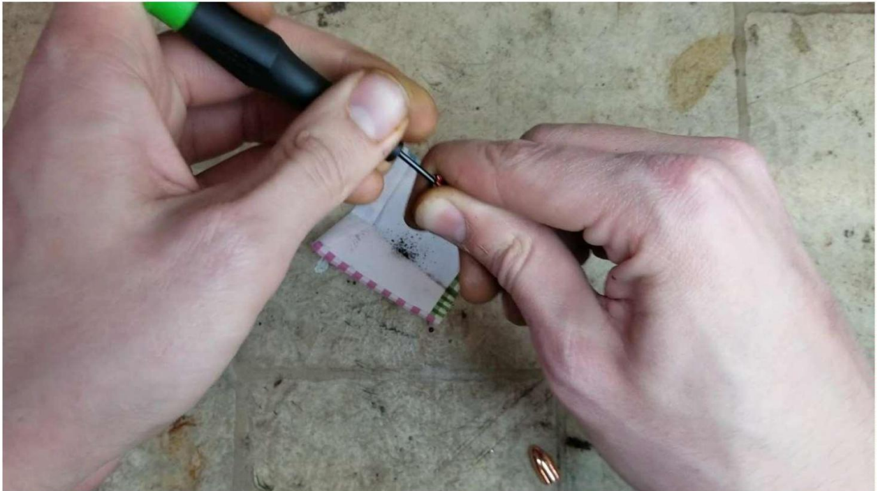
Step 6: Scraping the compound out of the Hilti
