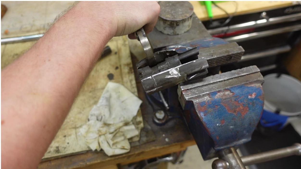
After grinding around the spot welds, peel the receiver stub off the trunnion with pliers.
